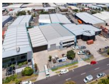
46 Andrew Baxter Drive Airport Corridor, Auckland
