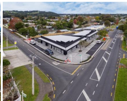
1047-1049 Coatesville-Riverhead Highway Riverhead, Auckland
