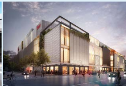
WESTFIELD NEWMARKET - REDEVELOPMENT, NEWMARKET UNDER CONSTRUCTION | 88,150m 2 (GLA)
