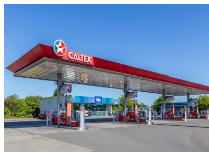
Two Caltex Service Stations Christchurch | $8,600,000
