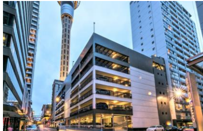
65-71 Federal Street, Auckland CBD Auckland | $40,000,000
