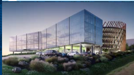
55 CORINTHIAN DRIVE, ALBANY UNDER CONSTRUCTION APEC PROPERTY DEVELOPMENT
