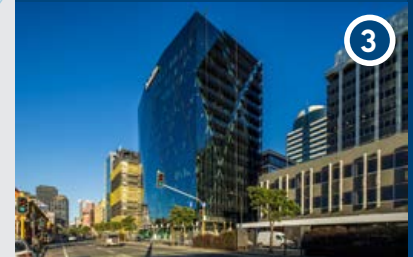
DELOITTE HOUSE, 20 CUSTOMHOUSE QUAY, COMPLETED | 17,000M 2 | Q2 2018 | NEWCREST AND WILTON CAPITAL
