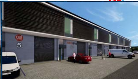
3-5 ORACLE DRIVE UNDER CONSTRUCTION MATVIN GROUP
